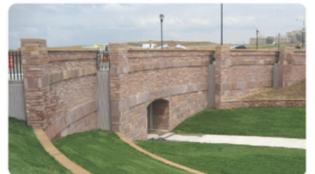
RidgeGate Parkway Underpass
