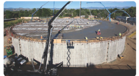
Ashland Reservoir Tank Replacements
